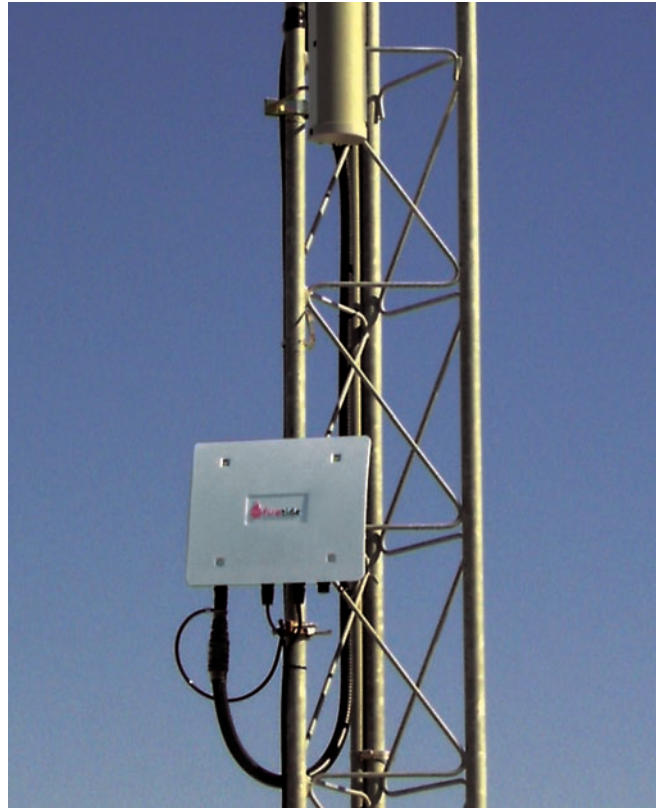
Firetide mesh node provides remote connectivity
