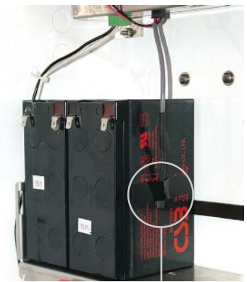
Tape Sensor to Battery
